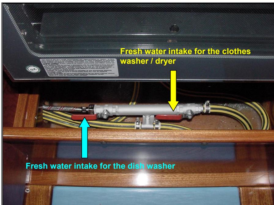
*Pict. 130 – Fresh water intakes stop cocks for the clothes washer / dryer and dish washer (photographed open)*
