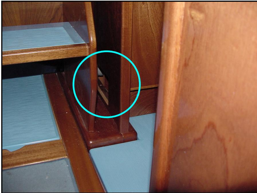
*Picture 75 – Refrigerator's air intake*
